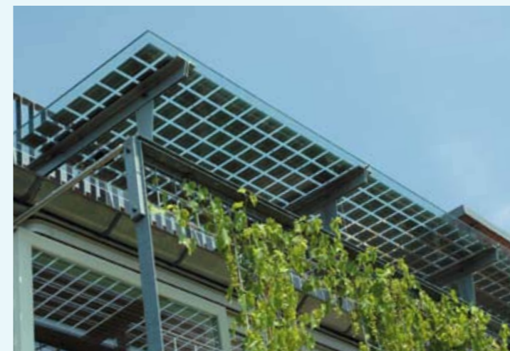
Shading canopy with power generation solar panels in Solothurn (CH).
