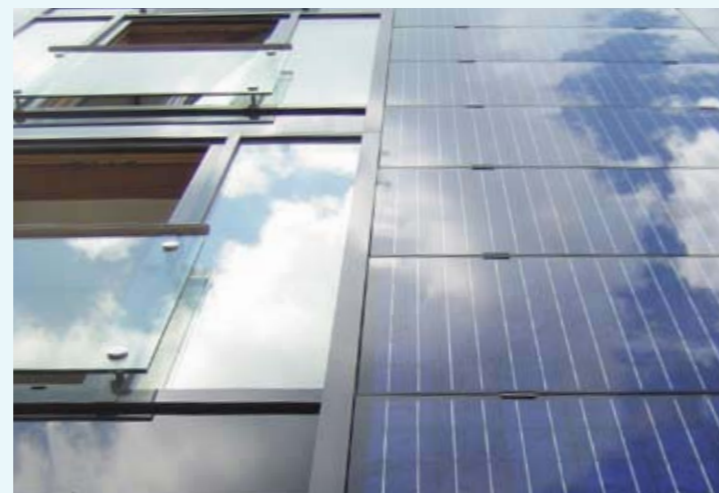
Custom 3S Swiss Solar Systems solar laminates for full facade integration in Landsberg (D).
