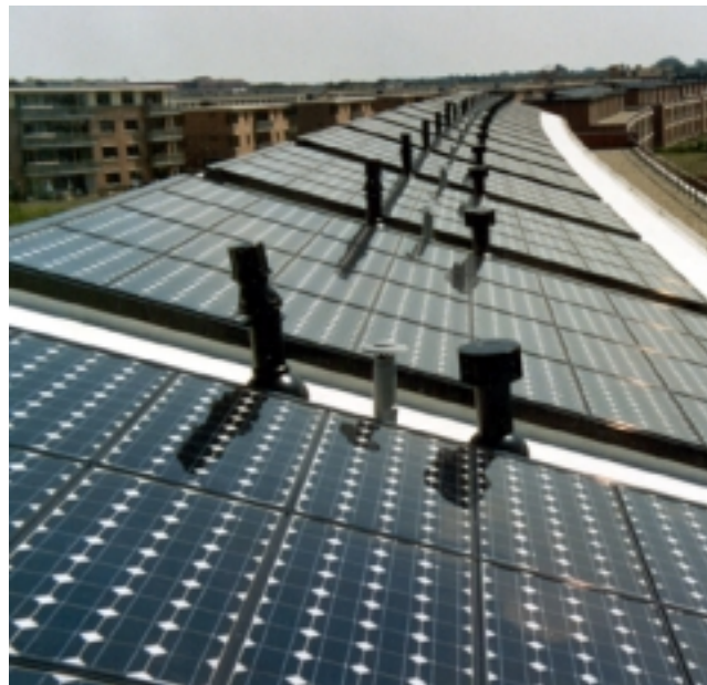
Photo 3: Roofs of Housing Scheme at Amersfoort, Holland
